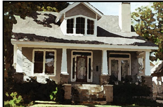
✓ Simple, raised stoop and a rhythm of piers with columns based on historically accurate details for the house style provide a sense of enclosure.
