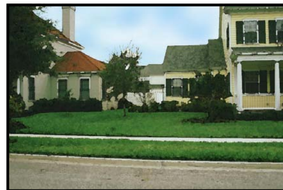
✓ These homes use wings to graduate a change in scale toward the abutting side yards.
