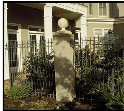
✓ This metal fence is articulated by masonry piers topped with finials.
