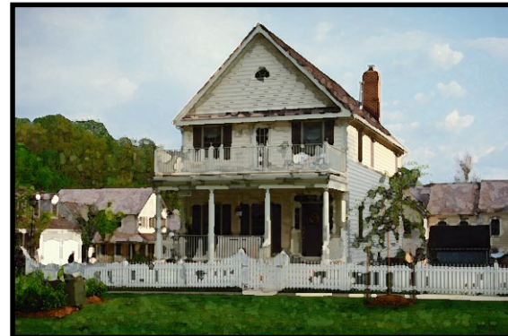
✓ By stacking a balcony on top of the porch, the house creates a more livable master suite, that can take greater advantage of views and its location facing a common open space.
