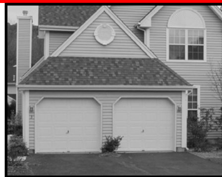
✗ Avoid inappropriately mixed roof forms, such as those that combine gables and hip. Various trim detail sizes create an irregular appearance.
