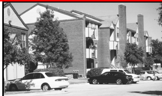
✗ Blank brick walls, poorly defined entries and lack of design cohesion result in an unattractive building.
