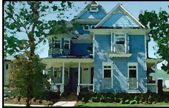
✓ Window details and the change in materials in the gables is historically based. Garage access is discretely to the side at the rear.
