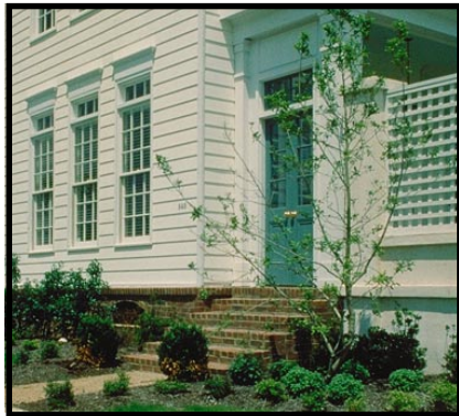
✓ This combination facade fence and wall encloses a side yard courtyard to the right of the home.
