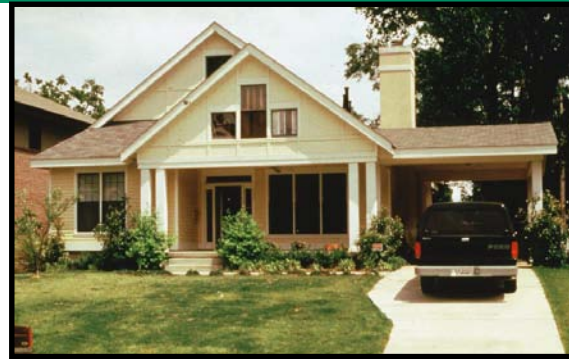
✓ A porte cochere can be used to provide covered convenience at a side door.
