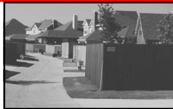
✗ The unfinished fences, unscreened utility meters and lack of landscaping create a barren appearance along this alley.
