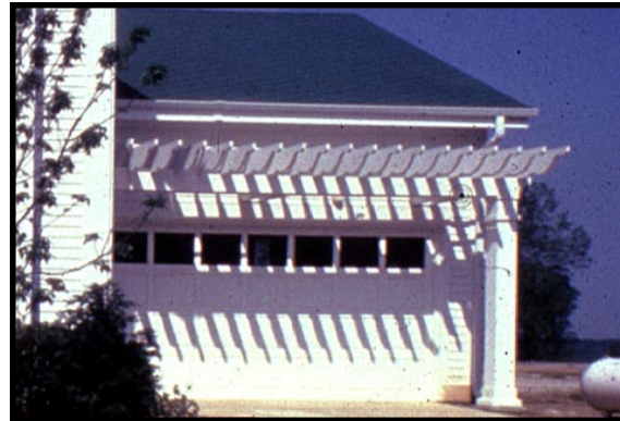
✓ Front access garages shall be recessed behind the primary facade and shaded by a minimum 2'-0" overhang or trellis.
