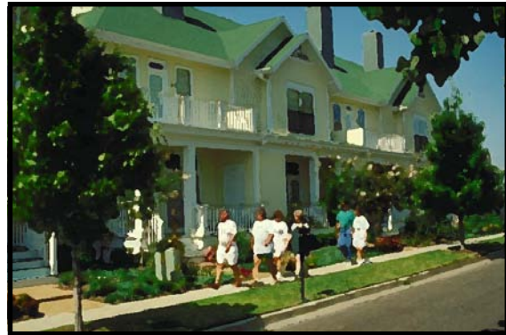
✓ Wall offsets, projections, recesses and changes in facade height are used to add interest and variety of this building.
