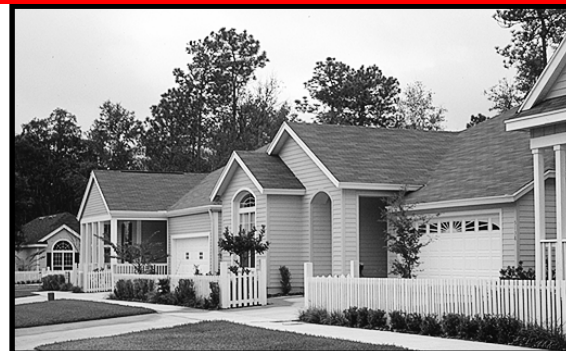
✗ Front garage extends forward off main entry, and oversized single garage door facing street is inappropriately detailed. Scale of main body is poorly defined by projecting gable end.
