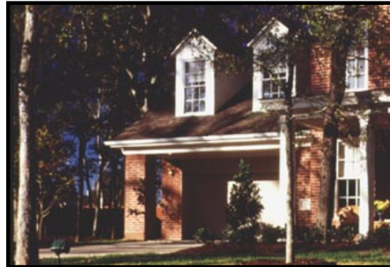
✓ Recessed garage doors are less visible when shaded by a deep roof overhang.
