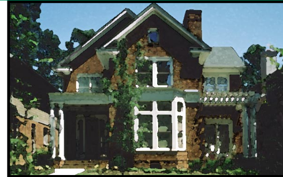
✓ The bay window seamlessly integrated into the forward gable, is balanced by a porch and pergola to achieve a richly detailed composition. Note the eave and rake details.
