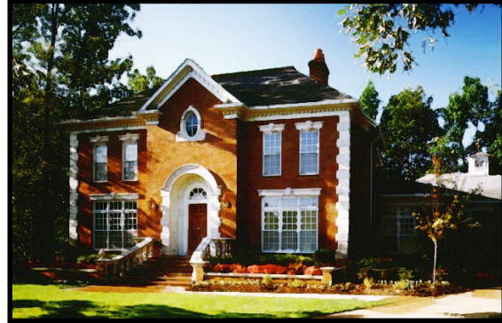
✓ This simple mass is accented by a projecting central bay containing a well-detailed arched entry.
