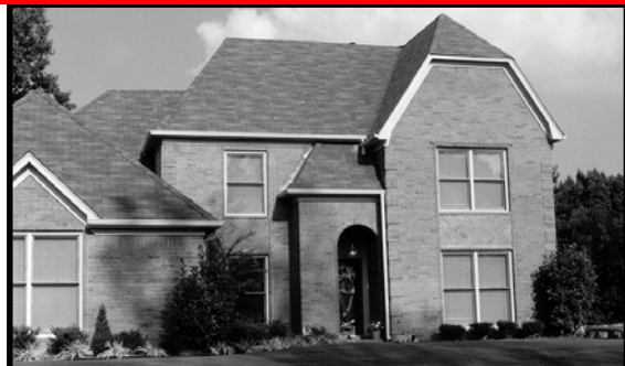
✗ Overall proportions are awkward. Roof mass, front entry, window heads and trim, cornice details, finish floor level, and brick quoins are all inappropriate.
