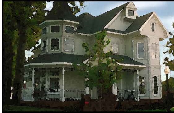
✓ This Victorian-inspired home responds to its corner location with a wrap-around porch and turret.
