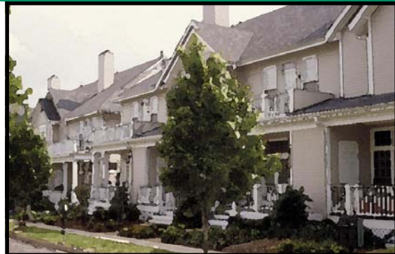
✓ Simple, overall massing roof form with appropriately spaced cross gables that add interest, consistent porch elements, and foundation planting.
