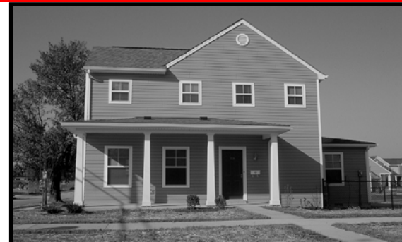
✗ This house is lacking a base and a proper cap along the top of the gable. The upper floor windows are undersized, resulting in too much wall in relation to window openings.
