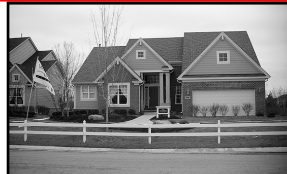
✗ The single prominent garage door, complex roof forms, and gable with columns on only one side result in an inappropriate composition that is costly to construct.
