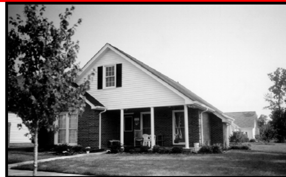
✗ Finish floor level is at grade and the porch columns are inappropriately scaled and detailed.
