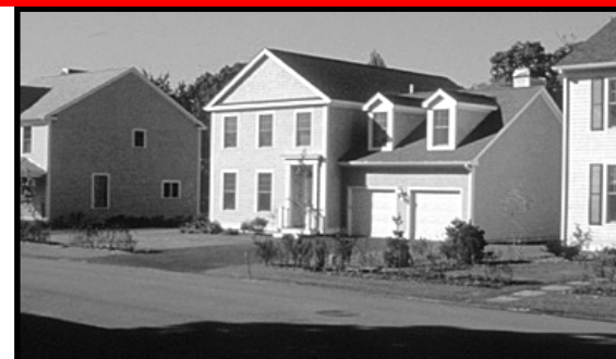
✗ While many elements are appropriate, the garage face is not recessed far enough behind the main body of the house. The neighboring sidewall to the left could also use more articulation.
