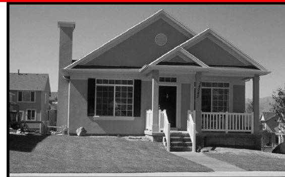
✗ Narrow shutters on double window, overly narrow staircase entry, and transom size are inappropriate details. Note the lack of foundation plantings.
