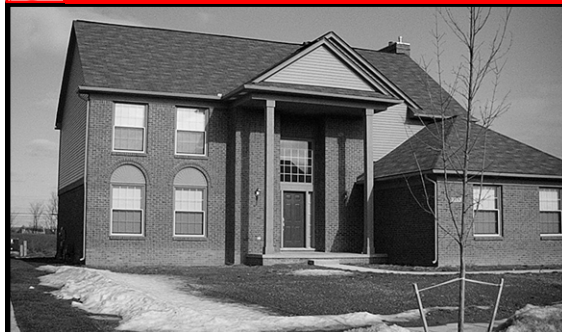
✗ The pediment is out of scale with narrow posts in the wrong location. The garage mass protrudes in front of the main body of the house.
