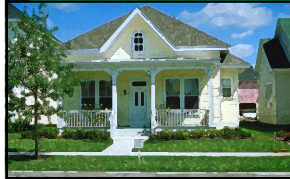
✓ Appropriate, simple design, properly utilizing one-story design fundamentals with raised finished floor level.
