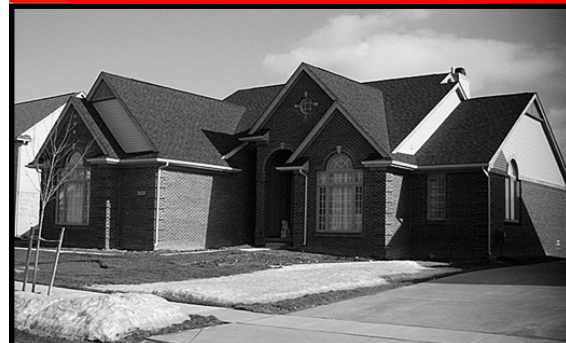
✗ The front entry is buried amidst a series of cascading rooflines and protruding gables, resulting in inappropriate massing and roof form that is also unnecessarily costly.
