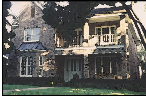
✓ Tall windows and doors with raised porch beam height provide appropriate vertical scale to the two-story veranda.
