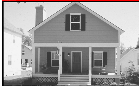
✗ Ceiling and window head heights too low, inappropriate column, cornice and rake details; second floor mass overpowers wall height below.
