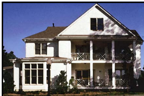
✓ Side porches can be combined with cross gable massing to achieve a diverse appearance from different angles along the street.
