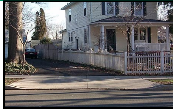
✓ This driveway is concrete between the street edge and the continuous concrete sidewalk; the remainder of the driveway is bituminous.
