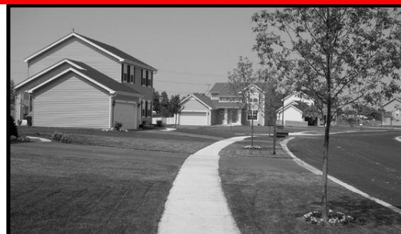
✗ This streetscape is characterized by too many blank walls and garage doors.
