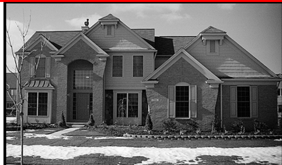
✗ This house is a confusing jumble of elements and details where each component screams for attention in relation to others. A simple composition is less costly.
