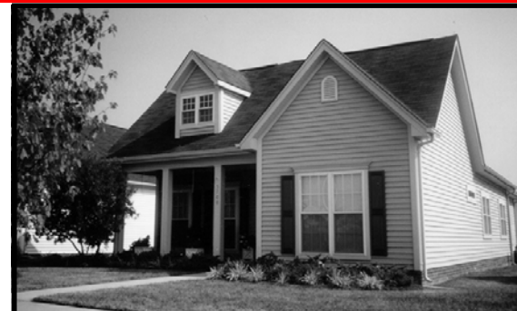
✗ Finished floor level and window head heights are too low. Shutters are inappropriate on a twin window and the dormer details are incorrect.
