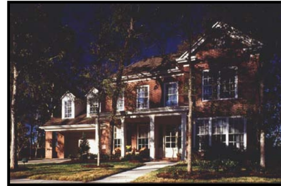
✓ A front-access garage steps back on the left side, but echoes the overhang and shadow effect of the front porch, which helps it blend into the overall facade composition.
