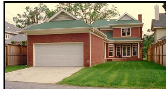
✓ This yard is enclosed and defined by the garage wing that extends to the alley. The garage complements the house, but is of a simplified design.
