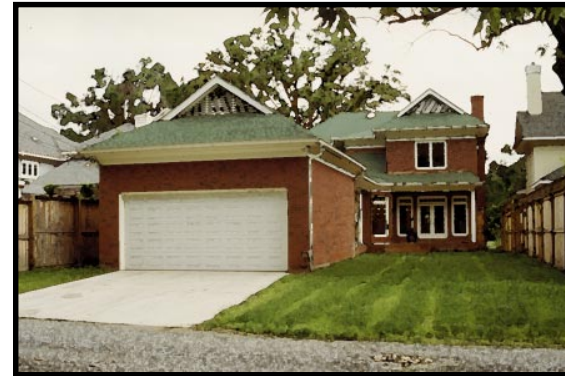
✓ Use of a garage form and materials that are compatible with the architectural quality of the home creates a sense of continuity. Note how the garage wing helps create a private rear yard.
