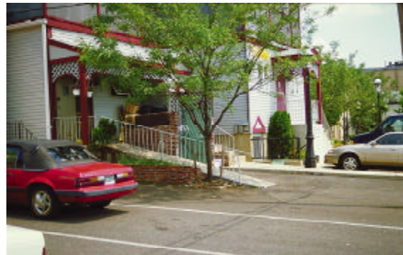
✓ This restaurant service area is incorporated into the body of the building in order to make it less visually apparent.
