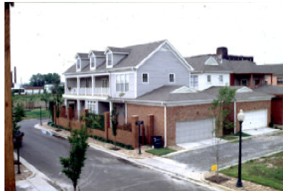
✓ The fence creates a nice street edge and allows for a private courtyard.
