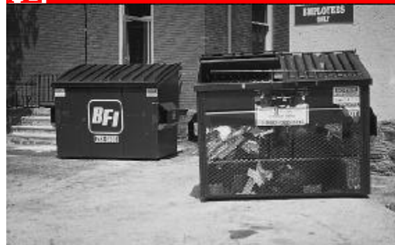
✗ Dumpsters and other service items should not be visually prominent and are required to be screened.
