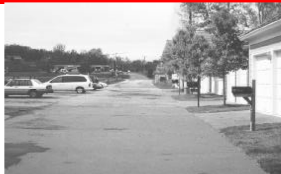
✗ Without landscape, there is a harsh transition between this parking area and the adjacent residences.
