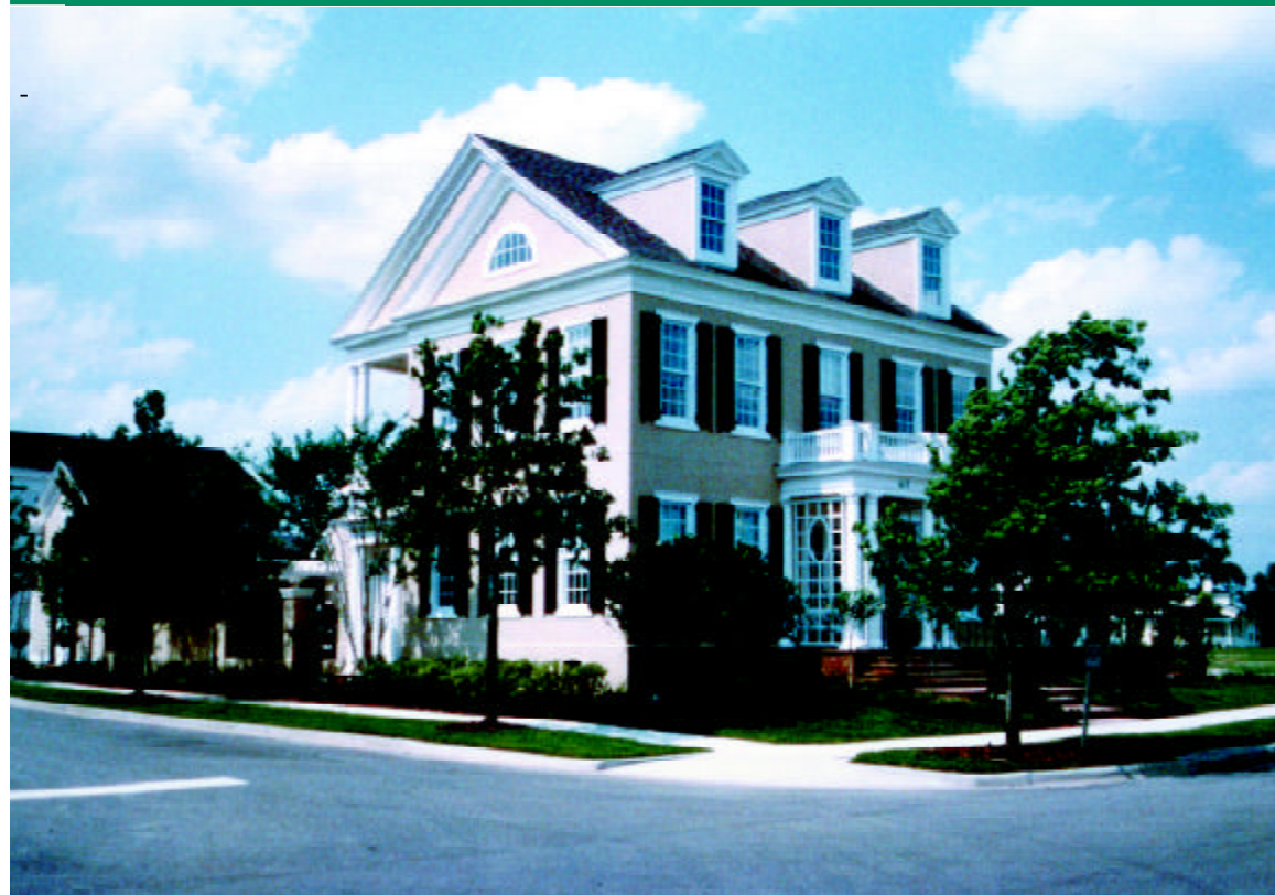
✓ Architectural character, materials and details continue from front to side, appropriately addressing both streets.
