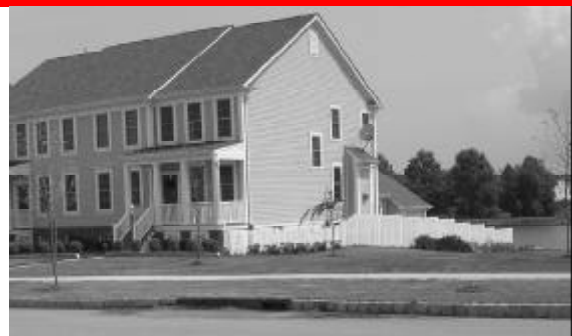
✗ The side of this home facing open space is inappropriately addressed with large amounts of blank wall, an unscreened direct vent fireplace and a visible satellite dish.
