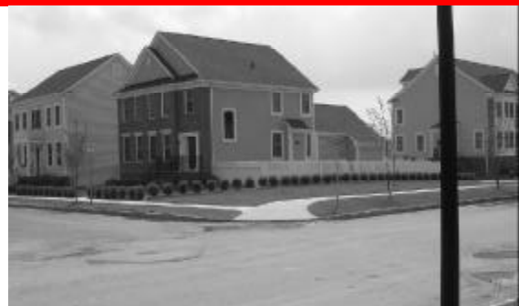
✗ While this corner lot has aligned windows and nice fencing, the brick does not return to a logical stopping point and the direct vent fireplace is not screened.
